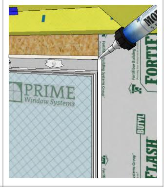
Tool the excess sealant squeeze-out flat before applying the side flashing.
