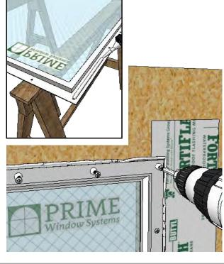
Cut 2 square pieces of SAF membrane material and apply them at each lower corner. Lay end dams upon the horizontal surface first, covering the flashing corner, then up the side trimmer of the RO. The material should extend outwards from the RO. Cut the lower edge of the material across the framing sill edge and swing the SAF out to the side of the vertical wall. J-roll the material flat. See drawing for additional detail. Ensure the SAF material at lower corners is tight at the inside corners.
